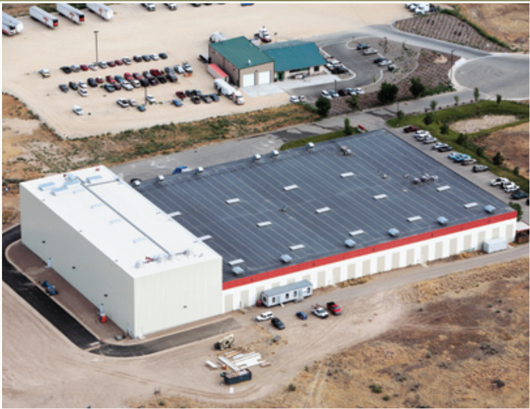
Liquor Dispensary Distribution Center located in Boise with 17,000 square foot expansion underway.
